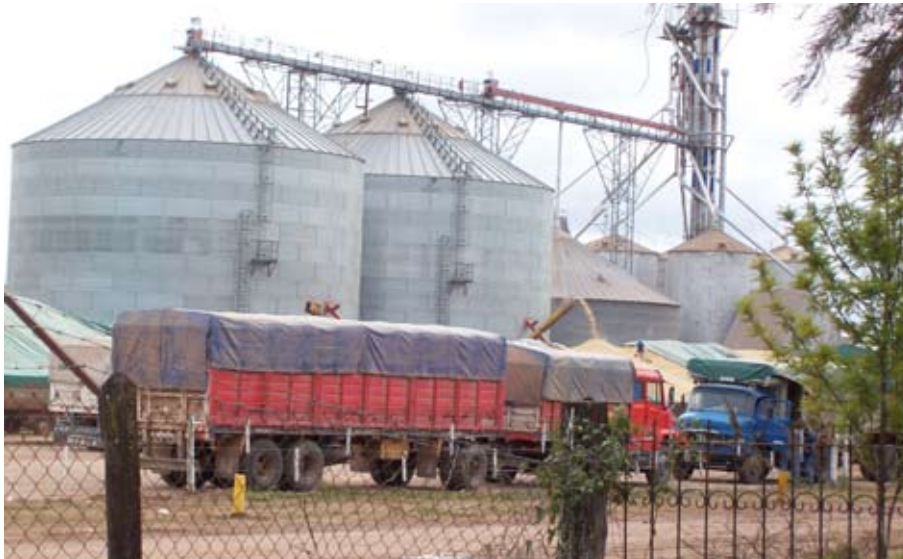
Bunge silos in the area of Las Lajitas, department of Anta, Salta
